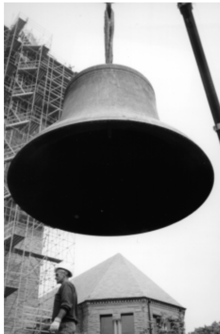
The Magna Marie, the largest bell, being removed from the tower
