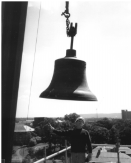
One of the bells being removed from the tower
