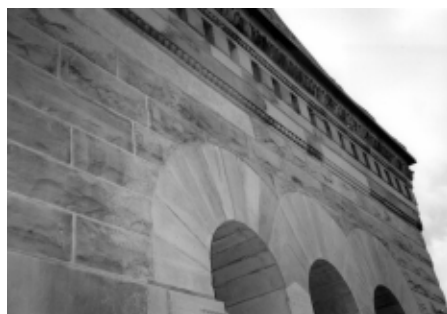
Retoiled arches and miscellaneous new stone
